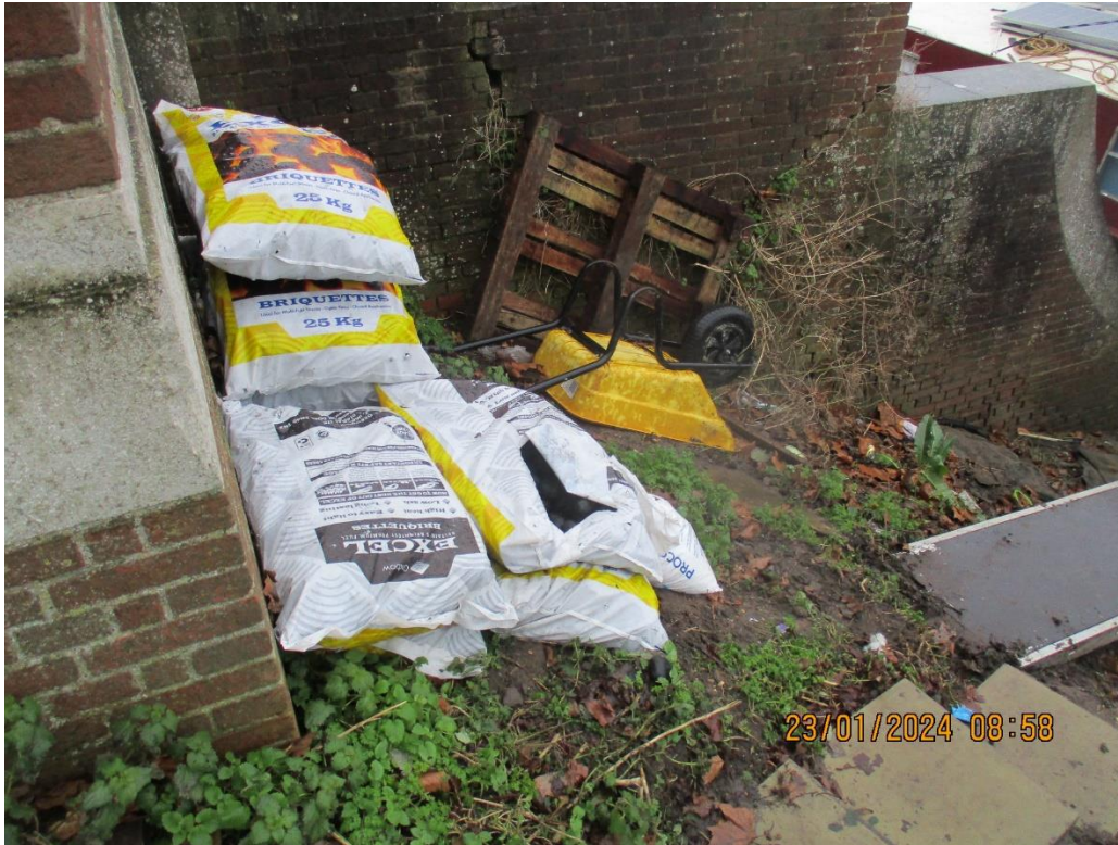
Picture 3 storage of charcoal, and installation of steps on EBC land without consent.
