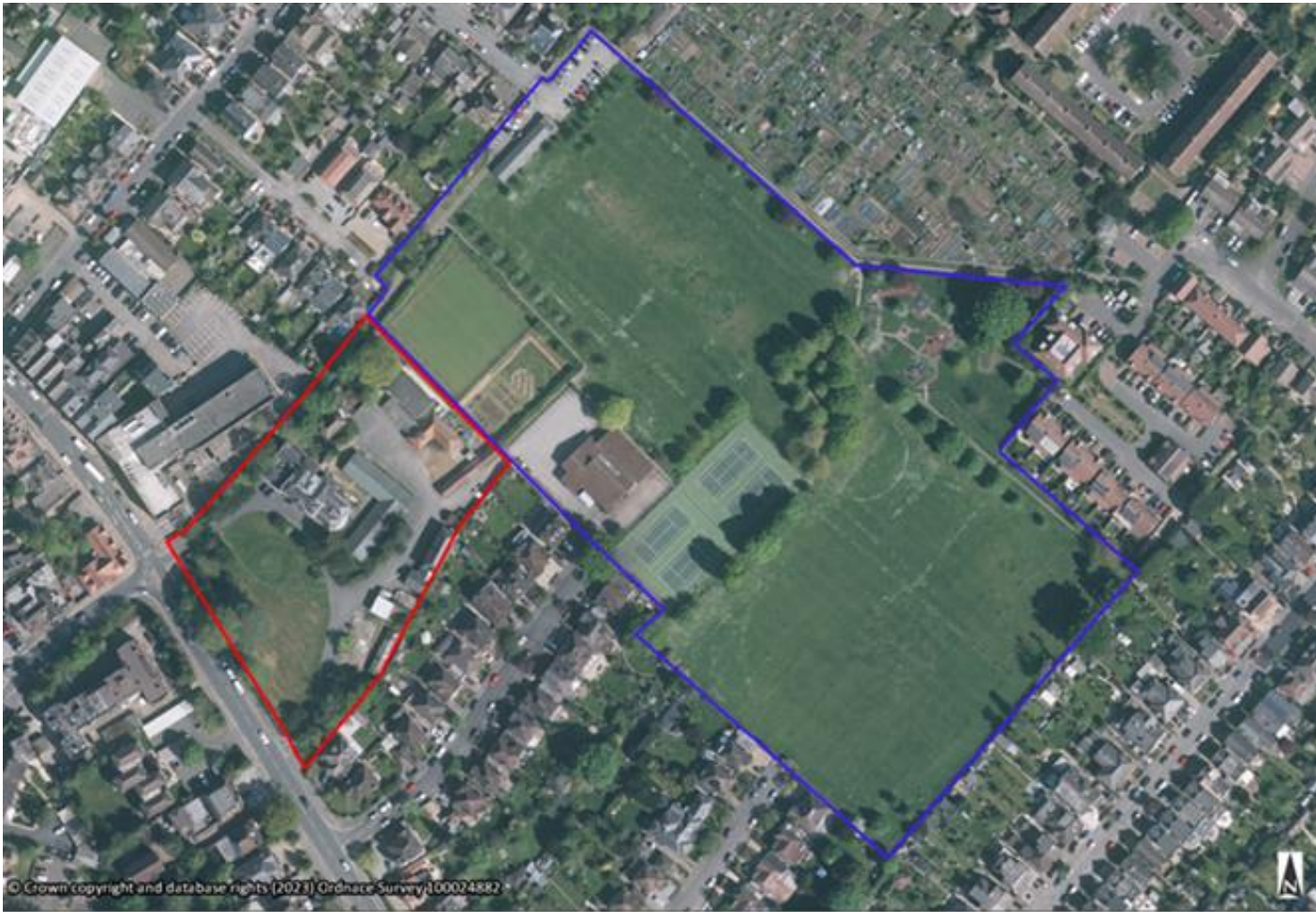
Figure 4: Aerial view of the existing buildings on Elm Grove (outlined in red) and facilities at Elmgrove Recreation Ground (outlined in blue)
