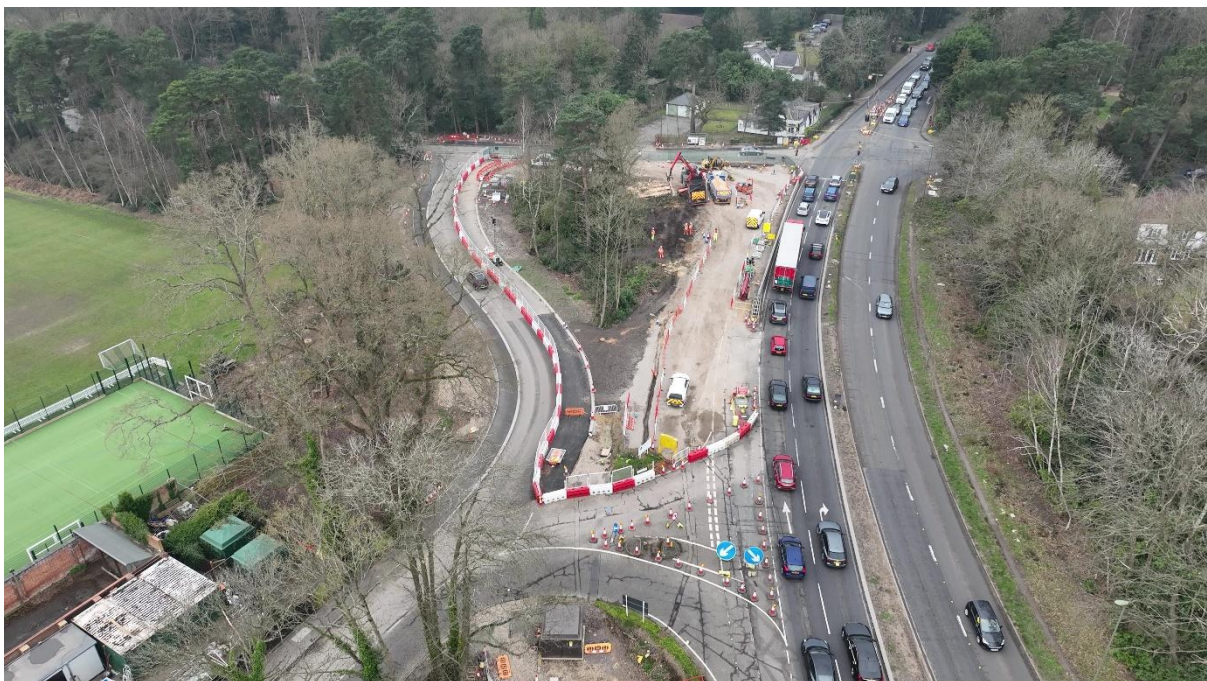
Figure 2: A245 on approach to Seven Hills Junction
