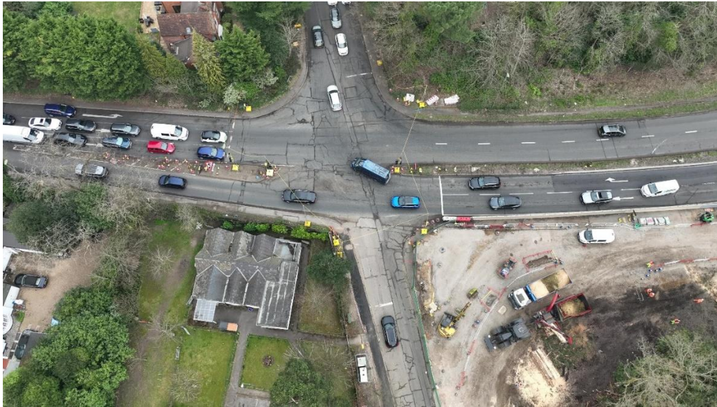
Figure 3: B365 Seven Hills Road Junction with A245
