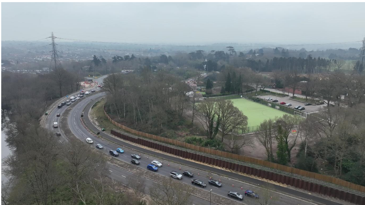
Figure 1: A245 on approach to Painshill Roundabout
